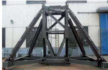
Ballast Chassis foundation
